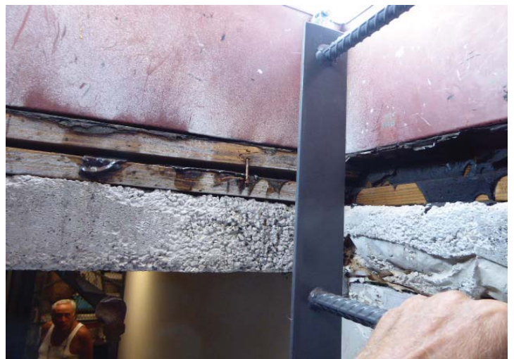
CEMENT ROOF VERIFICATION
